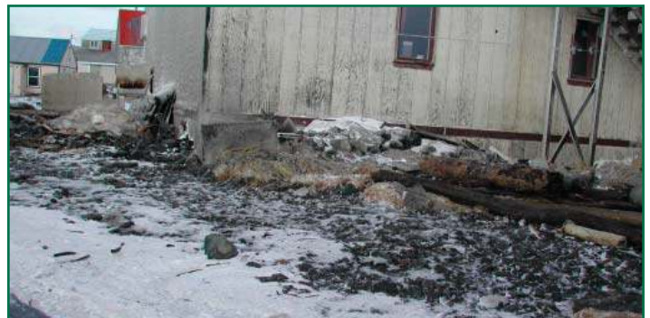
Flood debris by the Assembly of God Church.
