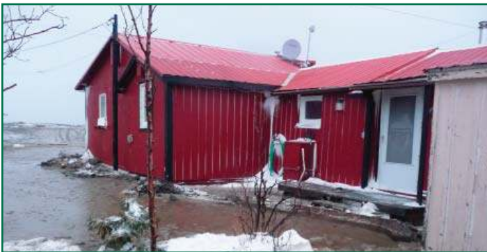
High water from the storm around Steve & Zoe Ivanoff's house in Unalakleet. You can see the dam they built to prevent the water from going underneath their home.
