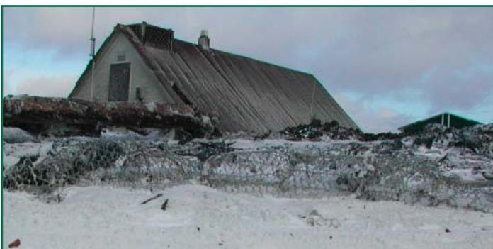
The storm water emptied the gabions in front of the 108 year old church. The gabions are wired mesh that are filled with rock to help protect the land from water damage.
